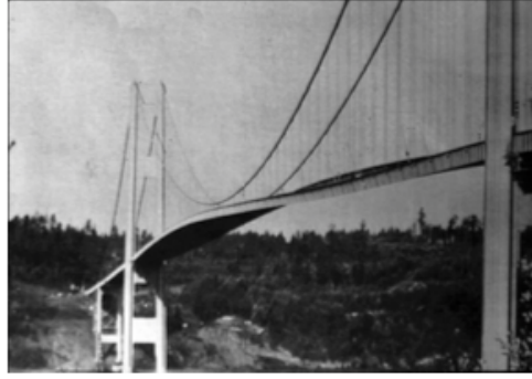
FIGURE 9.32. Photographs of the Tacoma Narrows Bridge prior to failure.
