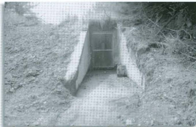
Once a carefully concealed and highly secure bunker, the Harbor Defense Command Post (entrance shown here) has been vandalized, as have many other former coastal defense sites. May 1998. (U.S. Army Corps of Engineers)
