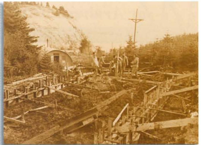
Construction of Quonset hut on Buskin Hill. March 1943. (Kodiak Historical Society)
