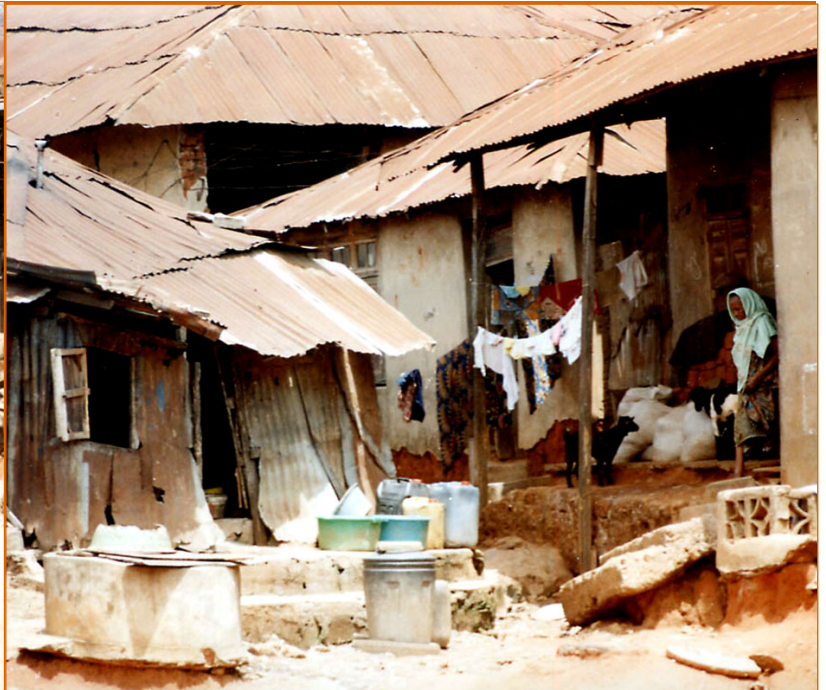
Photo 6 : Derelict houses in Bere
