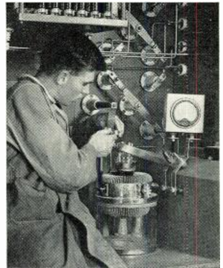
One of the high-powered tubes used in the new short-wave transmitters of "Radio New Zealand" at Titahi Bay, New Zealand.
